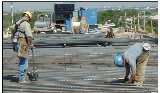
Figure 1: Rebar tying using a rebar tying machine (left) and manual tying using pliers (right).
